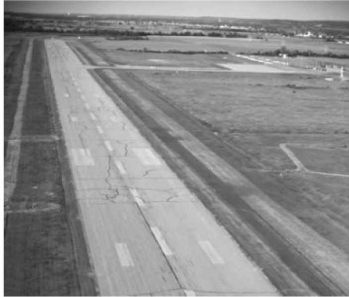
FIGURE C4.2.1(B) TYPICAL EXAMPLE OF TERRAIN CATEGORY 2 Excerpt from AS/NZS 1170.2 Supplement 1:2002
